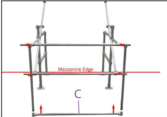
**12.** On opposite end to mezzanine edge insert part (C) horizontal tube by sliding tube 100mm up the vertical posts. Tighten using 1/4" hex key.
