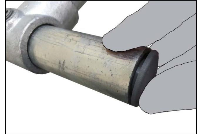
**14.** Place plastic end caps on all exposed tube ends. These may need to be tapped into place using a rubber mallet.
