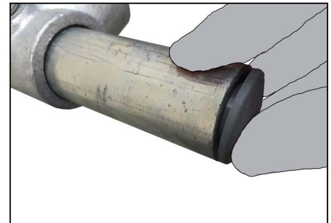
**11.** Place plastic end caps on all exposed tube ends. These may need to be tapped into place using a rubber mallet.
