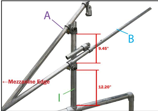
**6.** Carefully measure and mark 12.20" from top of frame as shown above. Slide part (B) onto part (I) and mount fitting at this mark, ensuring bearing is on the inside of the frame then tighten grub screw. Measure and mark 9.45" from top of fitting on part (B). Add part (A) to part (I) mounting the fitting to this mark ensuring bearing is facing same direction and tighten grub screw. Repeat process for other frame.
