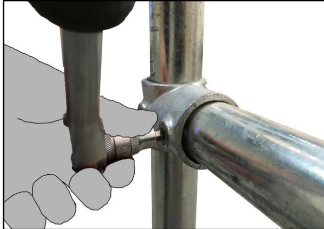
**13.** Ensure all fittings are correctly torqued to 39Nm and all tubes are level. Ensure gate operates smoothly and opens and closes positively.
