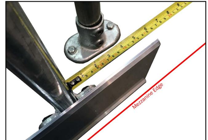
**11.** Check toe-board is central within the frame and tighten nuts to 15Nm to ensure it is held securely in place.
