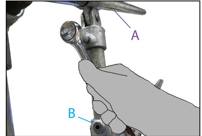
**8.** Connect cantilever tube link post form part (B) and connect into fitting on part (A). This will link the two tubes and allow the concertina action.
