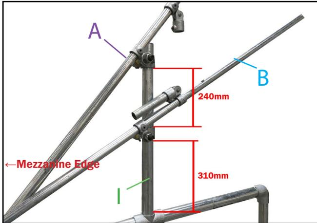
**6.** Carefully measure and mark 310mm from top of frame as shown above. Slide part (B) onto part (I) and mount fitting at this mark, ensuring bearing is on the inside of the frame then tighten grub screw. Measure and mark 240mm from top of fitting on part (B). Add part (A) to part (I) mounting the fitting to this mark ensuring bearing is facing same direction and tighten grub screw. Repeat process for other frame.
