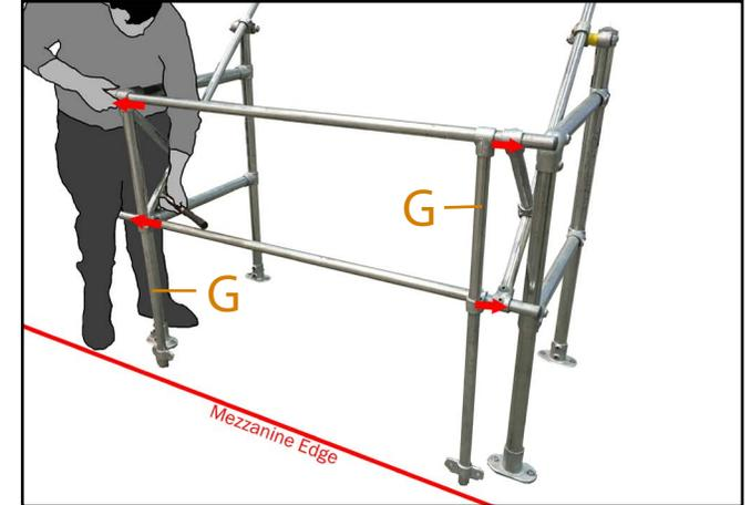
8. Slide part (G) vertical uprights to the left and right hand side of horizontals as shown above. Tighten using 1/4" hex key.
