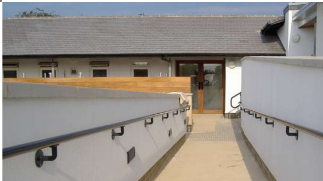
Right: ADA Compliant Railing for Access Ramps
