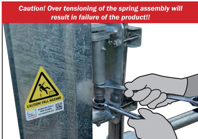
**M.** Once the gate is completely closed tighten the locking nut to hold the tension. Caution:- Continue to hold the ratchet firmly and do not release until the lock nut is tightened. Now remove the socket and spanner from the hinge. Repeat as necessary, to ensure that the gate closes sufficiently, once opened and released.
