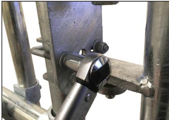
**D.** Torque all nuts/U Bolts to 39Nm using the 11/16" or 1/2" socket and torque wrench.
