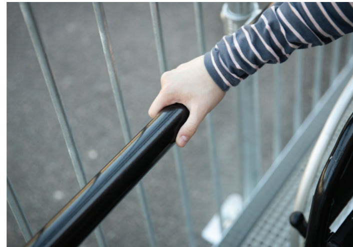
Handrail – Smooth, continuous, powder coated handrail that is not cold to the touch
